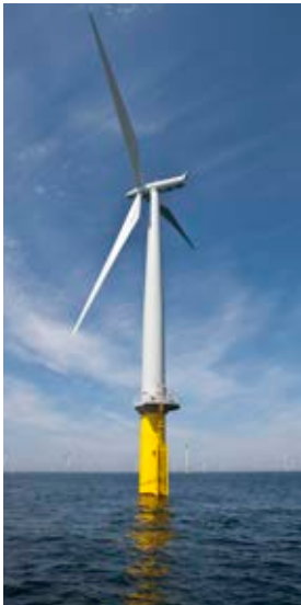
monopiles and transition pieces for offshore wind turbines
